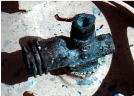
corroded Type 1 valve
