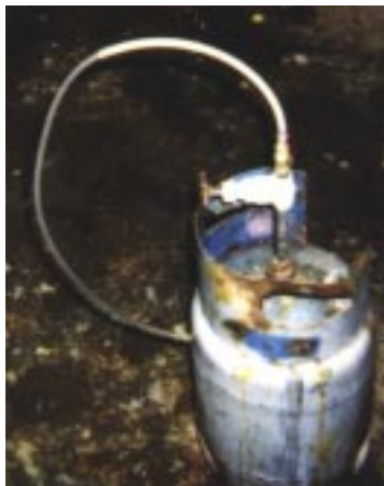
generator w/ hose
